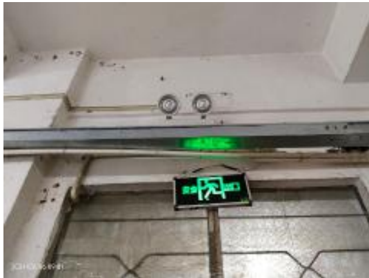
Safety exit sign and emergency lights.jpg
